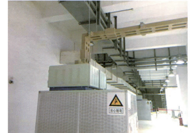
JDR与开关柜连接(上进) Connection with Switchboard(above)
