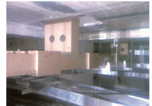
JDR与开关柜连接(下进) Connection with Switchboard(below)
